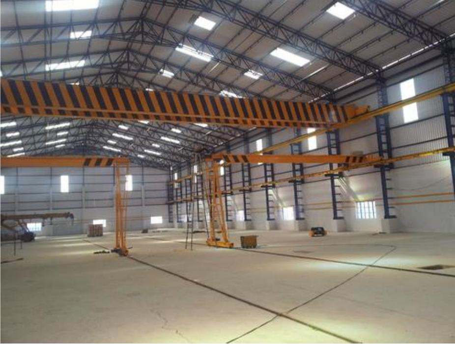
The goliath crane move on rails supported on floor level instead of rails placed at elevated level as in case of EOT Cranes. This eliminates the need for workshop building and hence reduction in capital cost. Goliath crane find major application in outdoors. However, the goliath cranes can also be installed inside a closed building.
